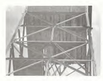
Figure 145. Details of bracing on the Coronado's Webb Peak lookout tower.
